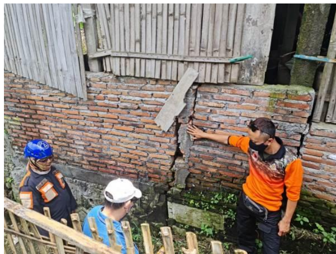
Figure 3: Cracks in the wall in the hamlet of Brau, Gunungsari village, Bumiaji sub-district, Batu city.
